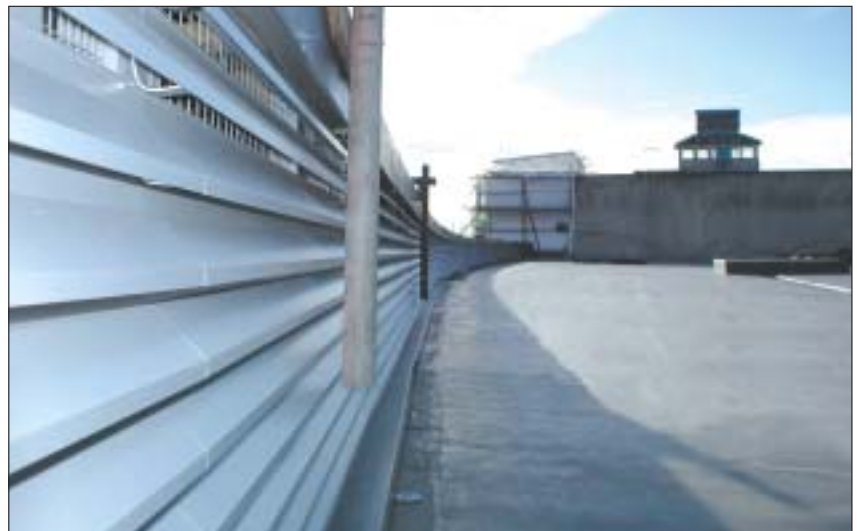
▲ Curved Louvre Screen installed at Kilcraigs Mill, Alloa.
