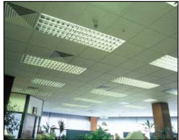
Louvre face diffusers in a typical installation
