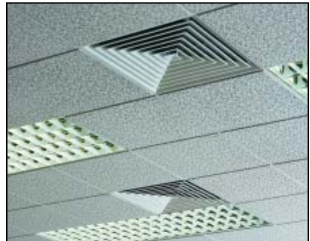
Louvre face diffusers in a typical installation
